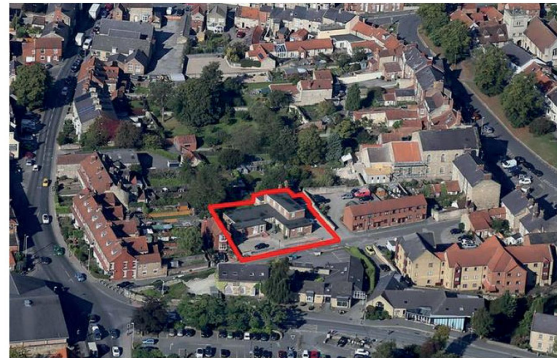
Aerial view of Pickering Health Clinic, Train Lane, site marked in red. Image: Alison Young
